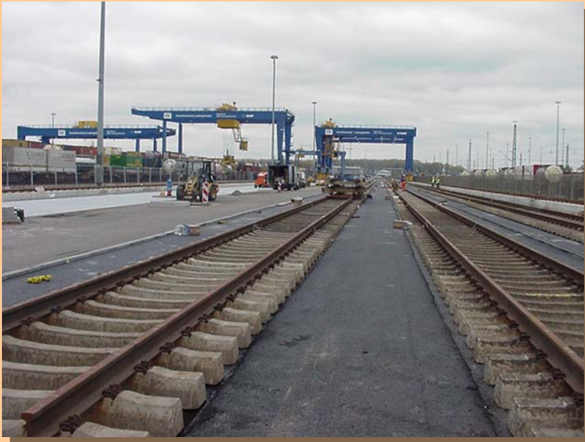
Wide-Span Crane Facility under Construction
