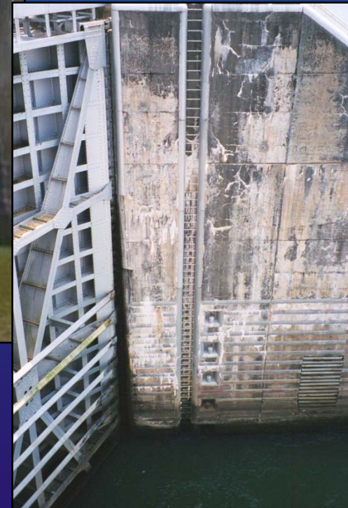
Concrete deterioration at Chickamauga
