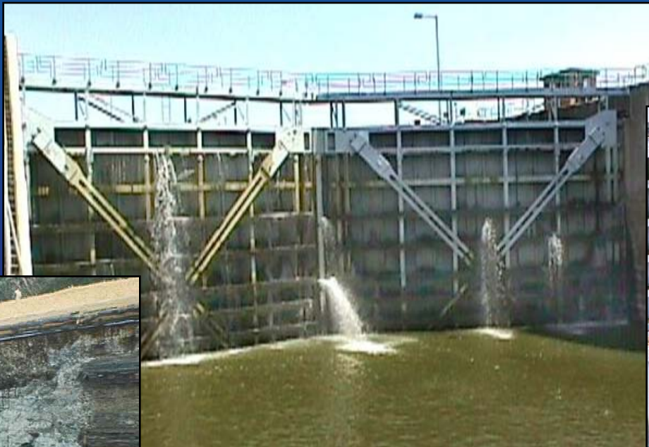
Leaking miter gates, Upper Miss Lock 19
