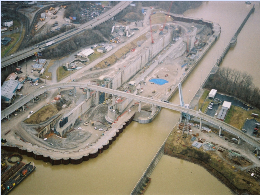
McAlpine Locks construction
