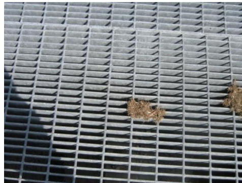
Figure 34 Current Conditions of Daylighting Grates Photo Credit: Stacy Cook
