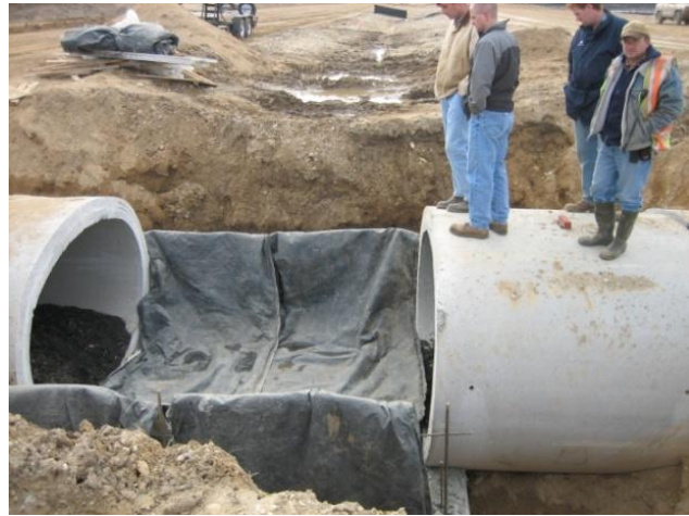
Figure 31 Installing Ecopassages Photo Credit: Gary Birch, WisDOT
