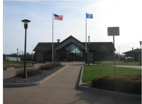
Figure 43 Wisconsin Rest Area #53 Photo Credit: Stacy Cook
