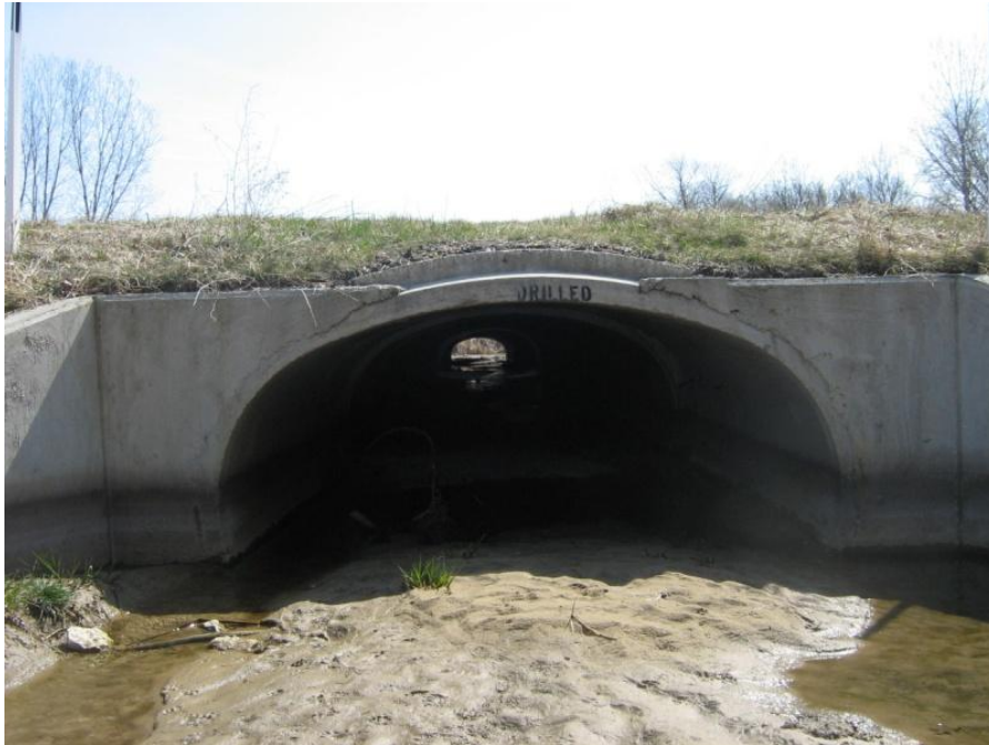
Figure 37 Current Conditions of Ecopassage Photo Credit: Stacy Cook
