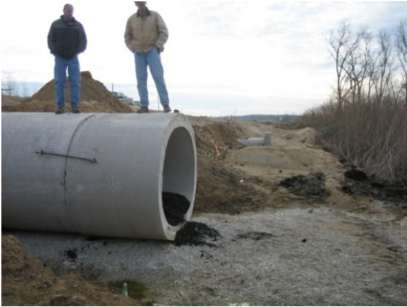
Figure 30 Installing Day lit Ecopassages Photo Credit: Gary Birch, WisDOT
