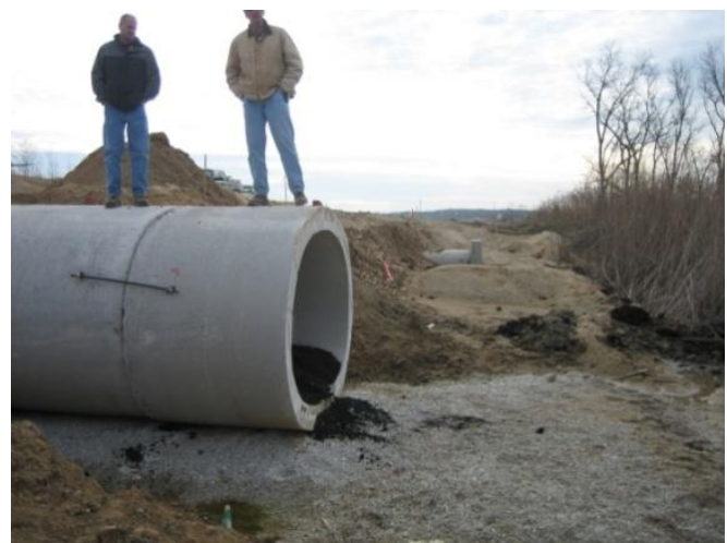
Figure 5 Installation of Ecopassage Photo Credit: Gary Birch, WisDOT
