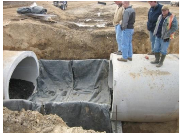
Figure 7 Installation of Ecopassage Photo Credit: Gary Birch, WisDOT
