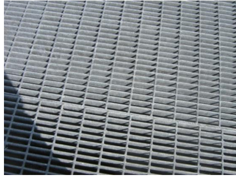
Figure 33 Current Conditions of Daylighting Grates Photo Credit: Stacy Cook
