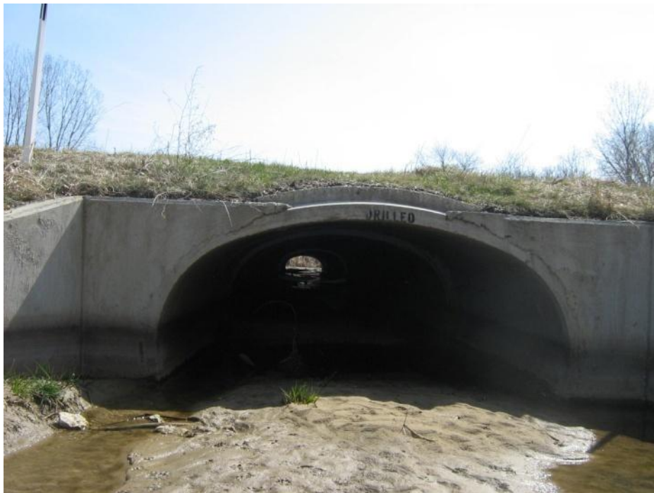
Figure 38 Current Conditions of Ecopassage Photo Credit: Stacy Cook
