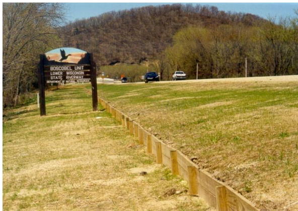
Figure 17 New Turtle Barrier Photo Credit: Bob Swartz
