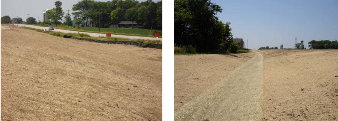
Figure 5. Slopes and Ditches Constructed with GPS Machine Guidance on Hoffman Project
