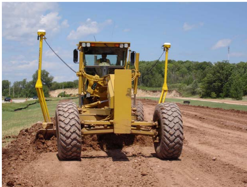
Figure 1. Hoffman Grader Mounted with Trimble GPS Machine Guidance
