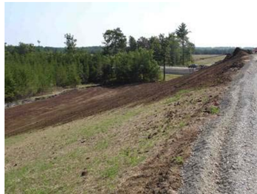
d) Finished Slope and Ditch
