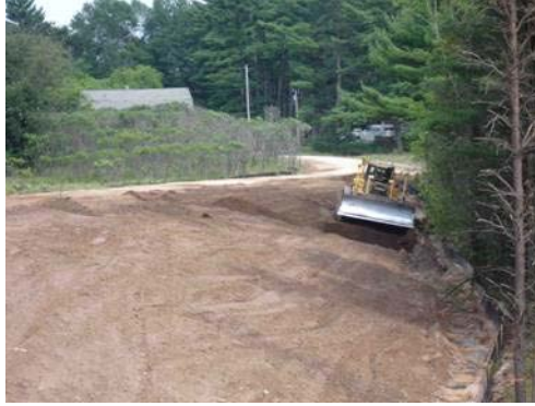
Figure 11. Dozer Spreading Topsoil on Steep Slope near Tree Canopy
