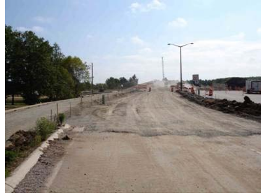
b) After Gravel Placement
