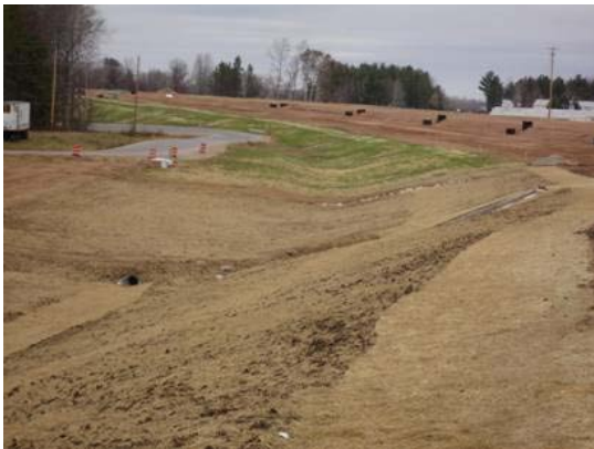
a) Finished Slopes and Ditch
