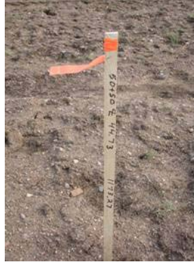
Figure 5. Kowalski Road Slope Stake Lath Marked with Station, Offset, and Elevation.
