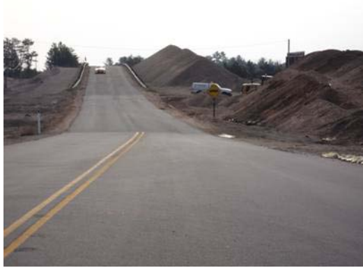
a) Prior to Construction
