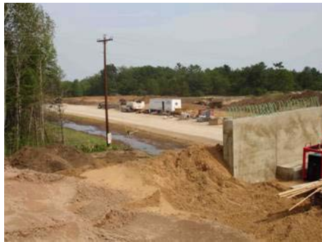
Figure 12. A Segment of Main Line Sub Grade that was Blue Topped because the Model had not yet been Reviewed.
