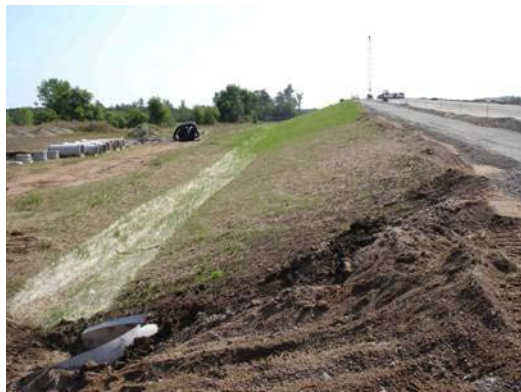
c) Finished Slope and Ditch
