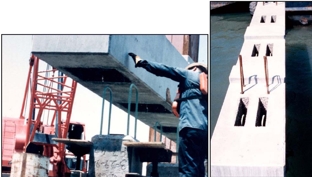
Figure 9 – Grouted Pocket Connection (14)
