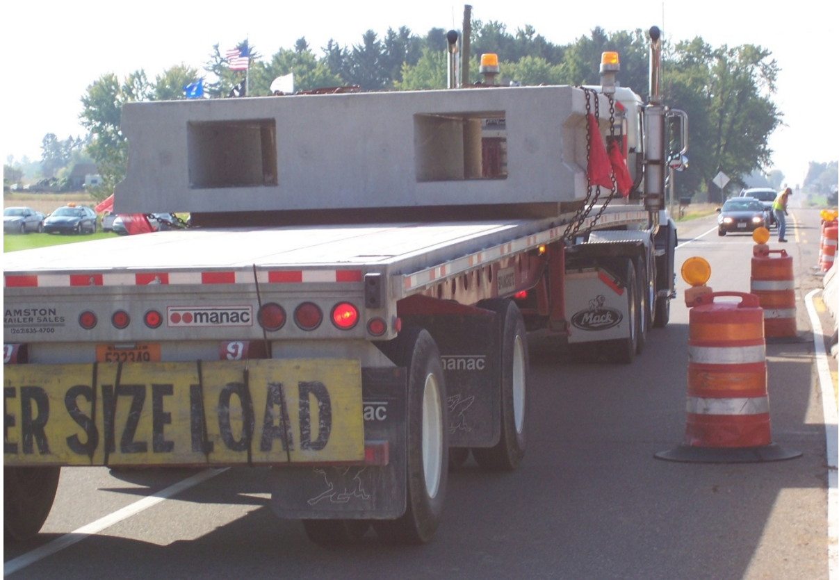
Figure 14 – Cross section of an abutment segment showing the voids left for pile placement and the female keyways at the edges.
