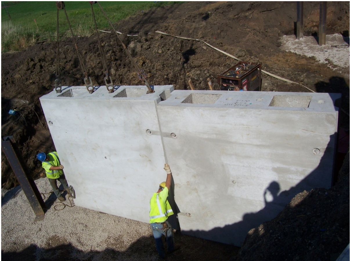
Figure 15 – Setting the second abutment module in place
