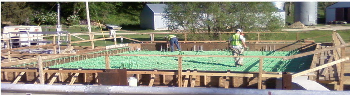
Figure 10. Rebar Installation of Structural Deck
