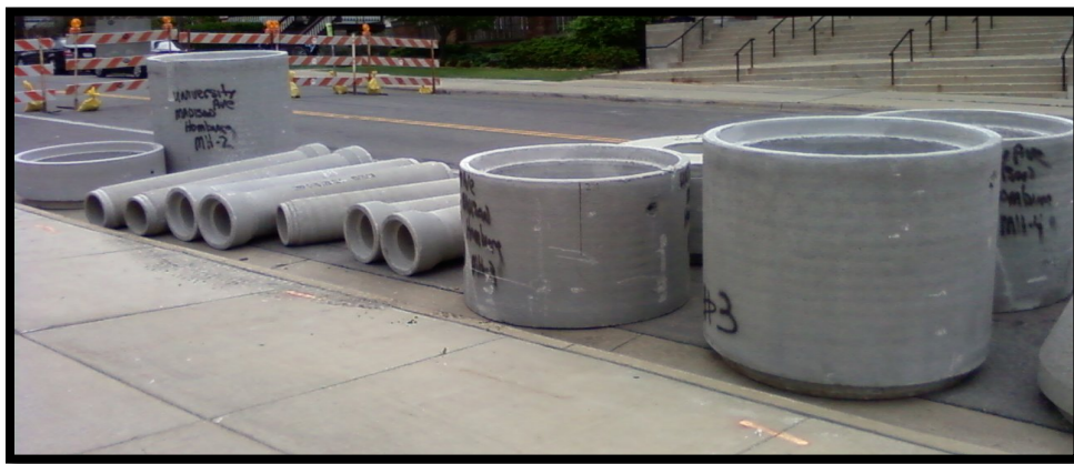
Figure 5. Example of Storm Sewer Waste
