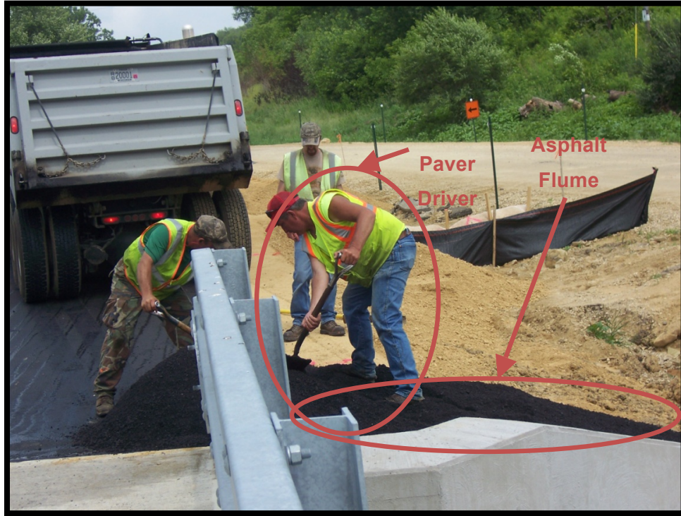
Figure 21. Asphalt Flume Picture 2
