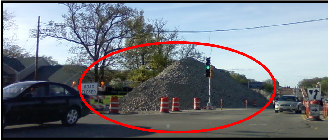
Figure 6. Illustration of Waste in Road Construction
