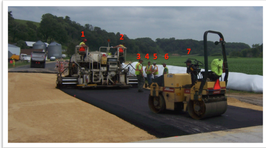
Figure 19. Crewmembers Waiting for Asphalt Truck
