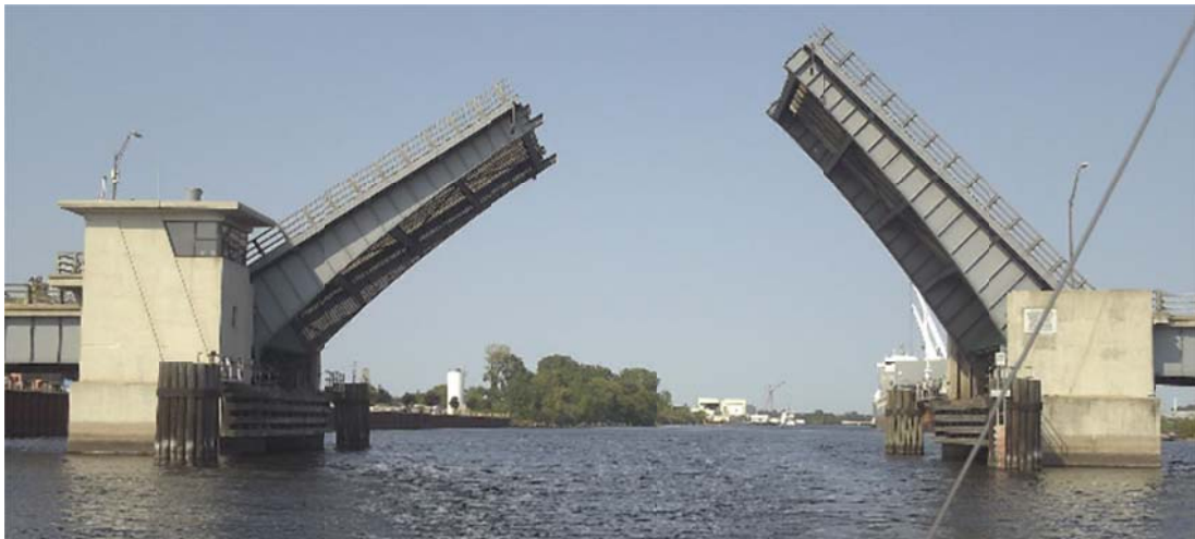
Figure 4.1-2. Marinette Bridge (Wisconsin, HIS ID: B38016, Bascule bridge, span = 143 ft.). Reprinted from BridgeHunter.com
