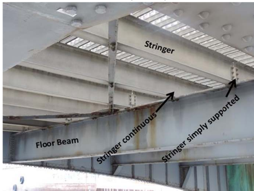
Figure 4.1-6. Marinette - alternate supports for stringers.
