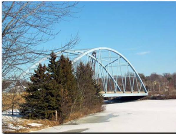
Figure 7.1-1. Chippewa River Memorial Bridge (Wisconsin, HSI ID: B-09-087)
