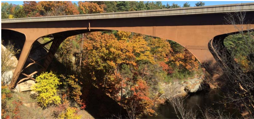
Figure 3-1.1. Mirror Lake Bridge (Steel rigid frame bridge, span = 324 ft.)
