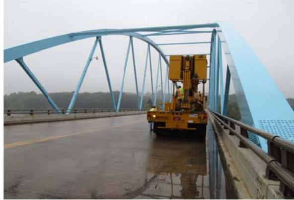
Figure 7.1-3. Chippewa bridge deck during inspection in 2013.
