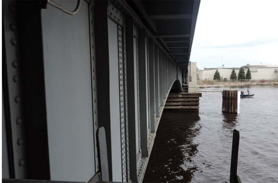
Figure 4.1-5. Basculer Girder view. Stiffeners every 3.5 ft. and a variable cross section along the bridge.
