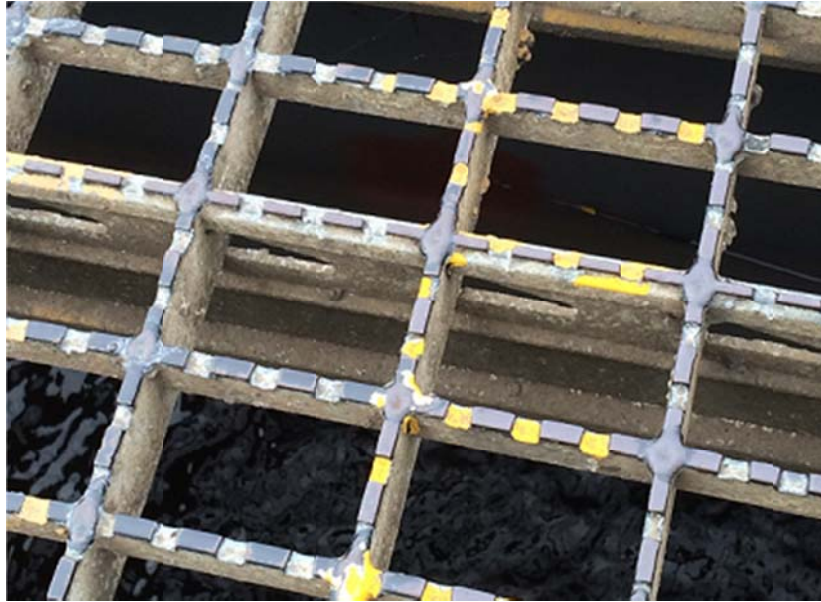
Figure 4.1-5. 5-in. steel open welded grid flooring.
