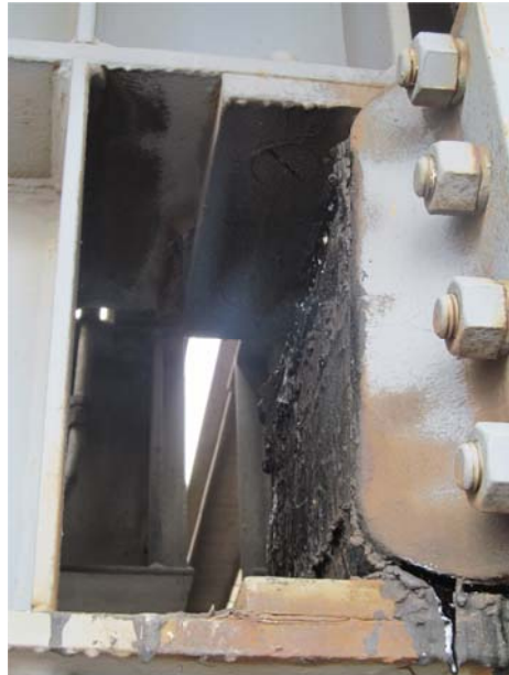
Figure 4.2-14. Joint between leaves of Marinette bascule bridge.
