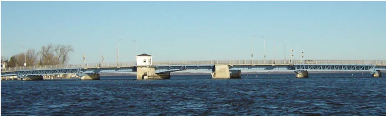
Figure 5.1-1. Winneconne Bridge (Wisconsin, HSI ID: B709130002, Bascule bridge, span = 95 ft.)
