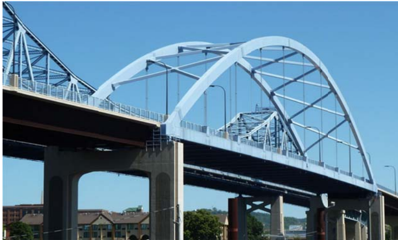
Figure 6.1-1. Cameron Ave Bridge
