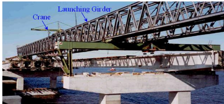
Figure 2.10. Launching Girder and Crane Operations in Bridge Construction
