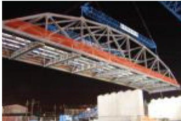
Figure 2.6. Preassembled Superstructure Installation
