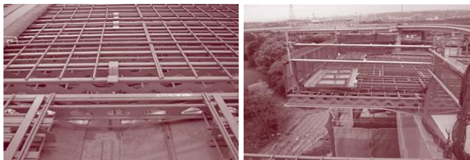
Figure 2.9. Hybrid Steel-Concrete Deck System
