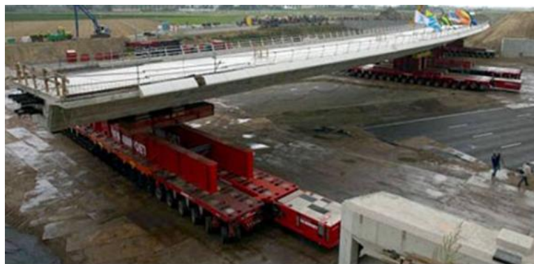
Figure 2.11. Preassembled Superstructure Installation Using Self-Propelled Modular Transporters
