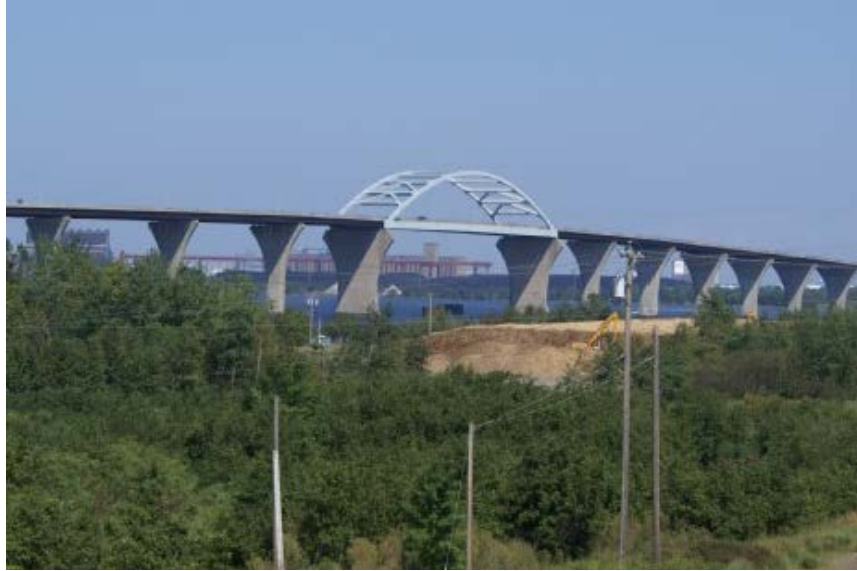
Figure 5. Bong Bridge (Wisconsin, Tied arch bridge, Span = 500 ft).
