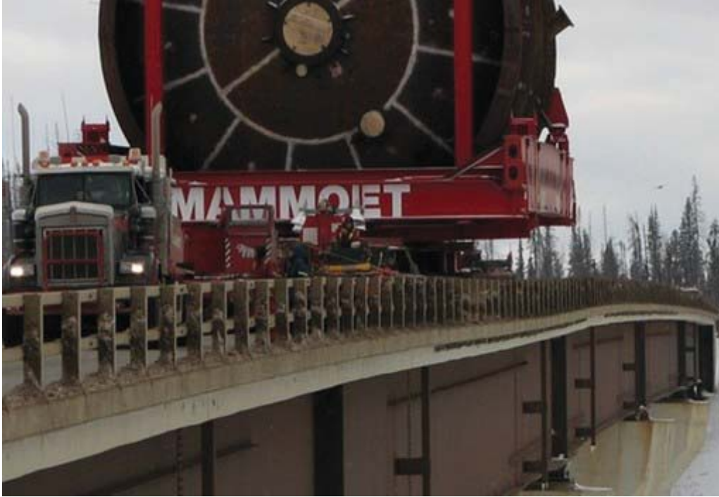
Figure 1.1: Overweight vehicle on a bridge (Foley, 2007)
