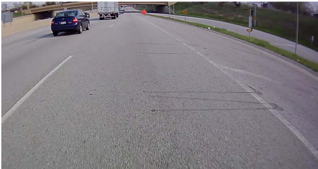
Figure 8.2: Wander and WIM Systems After 5-1/2 years of Trafficking
