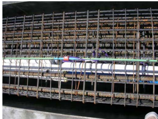
Figure 4.10: Installed Sister Bar Strain Gages (Abu-Farsakh et al. 2010)
