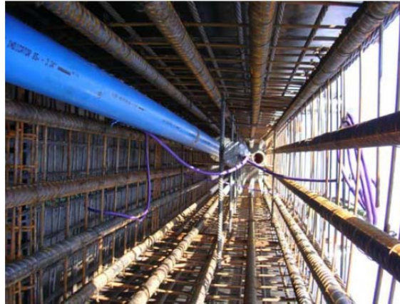
Figure 4.9: Installed IPI Casing (Abu-Farsakh et al. 2010)
