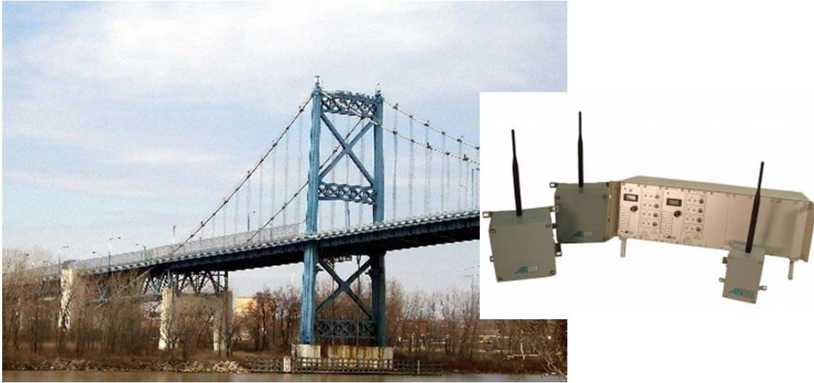
Figure 3.26: Implementation of a Wireless Bridge Health Monitoring Telemetry System (ATItelemetry.com 2011).
