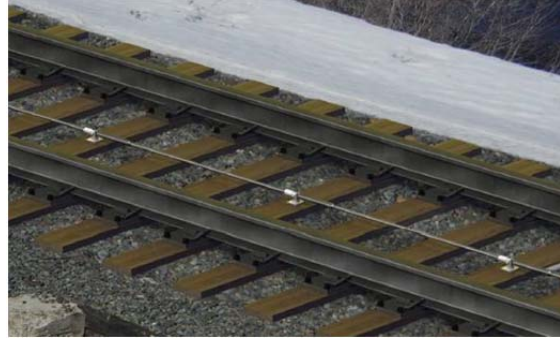
b. Settlement Sensors installed at a Railroad ( http://www.rstinstruments.com )
