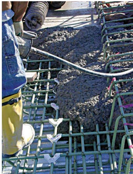
Figure 3.28: Installation of Smart Aggregate units (Carkhuff, 2003)
