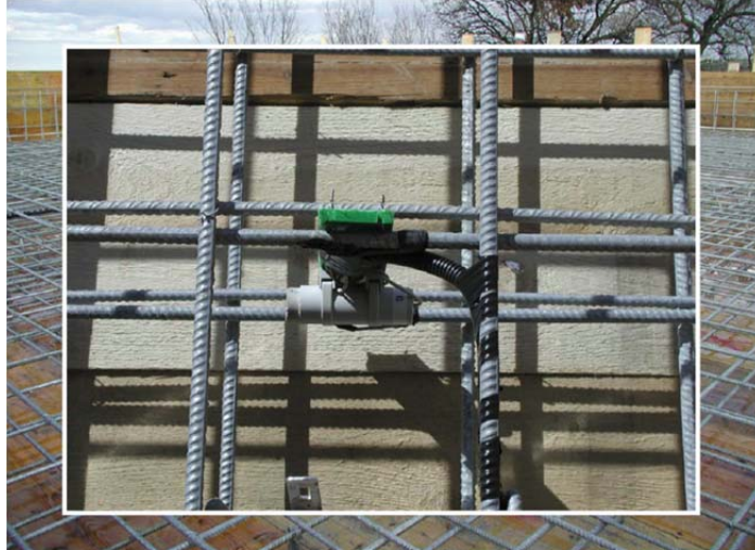
Figure 4.12: The installation of IRH sensor (Moriconi and Naik, 2010)
