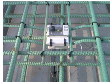
b. Installation of ECI corrosion meter (Virginia Technologies, Inc.).
