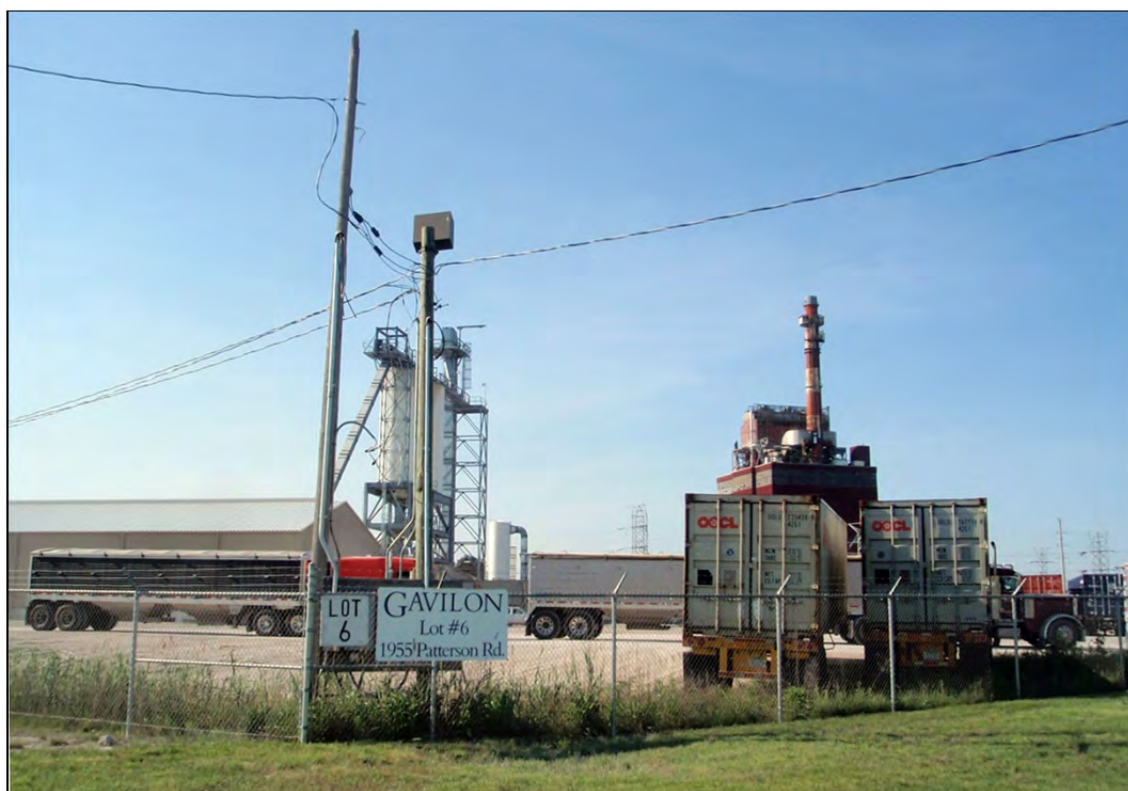
Figure 34: Gavilon Grain Transloading Operation (Photo: R.D. Stewart)
