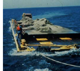
Open water placement
