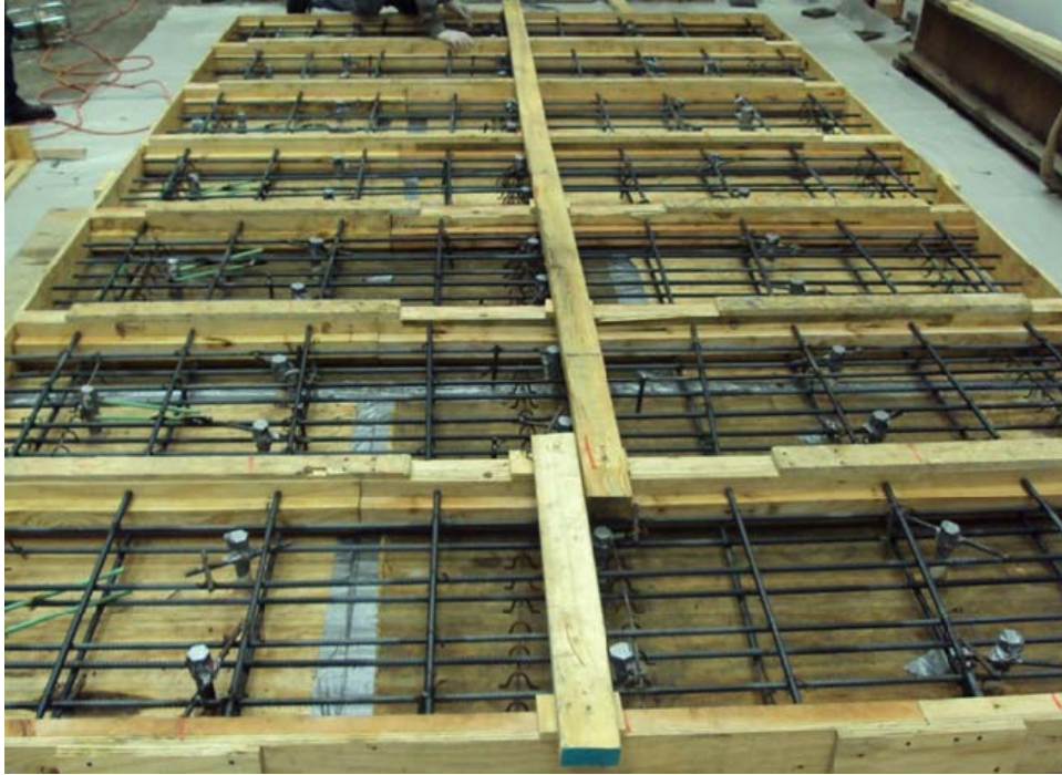
Figure 3.7: Reinforced Concrete Panels Form Work
