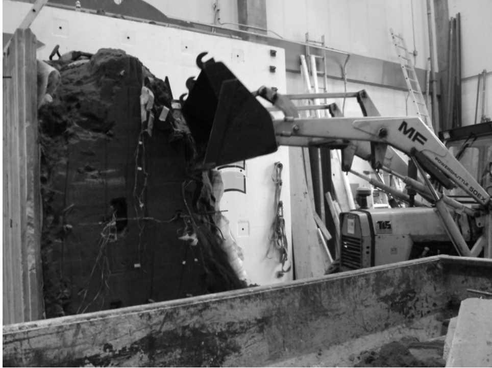
Figure 3.19: Excavation of the CLSM Backfill
