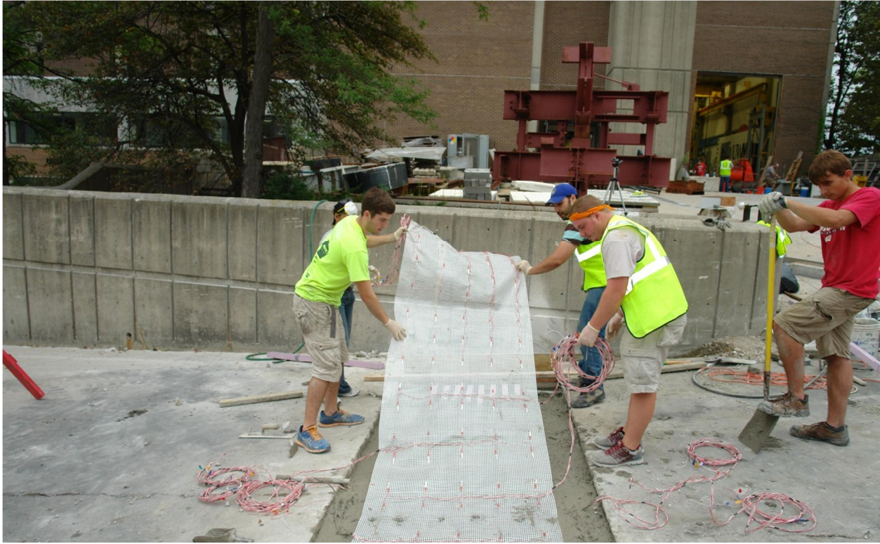
Figure 47: Placing of the PVA mesh on the slab
