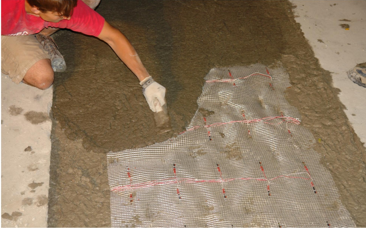
Figure 48: Placing the electrically conductive material on the SECC slab
