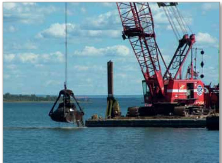
Dredging material off Erie Pier, Port of Duluth-Superior Photo credit: Wisconsin Sea Grant Institute
