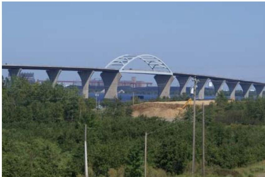
Figure 7-11. Bong Bridge (Wisconsin, Tied arch bridge, Span = 500 ft)
