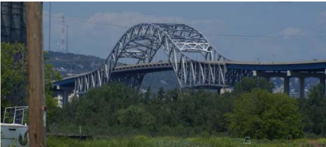
Figure 7-2. Blatnik Bridge (Wisconsin, Truss Bridge, Span = 270 + 600 + 270 ft)
