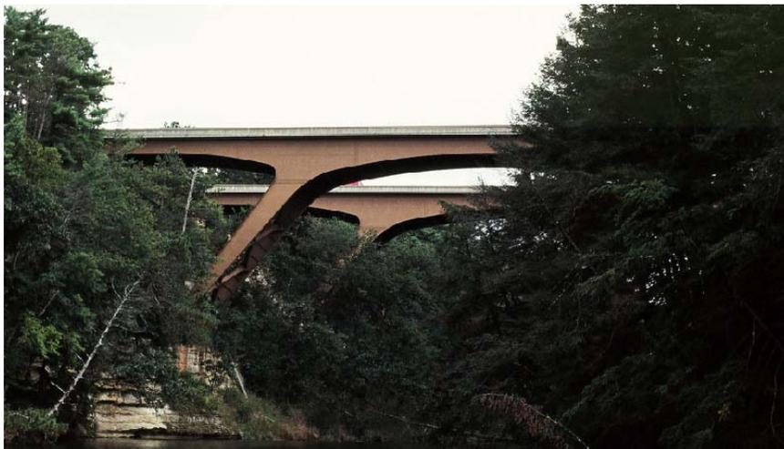
Figure 7-3. Mirror Lake Bridge (Wisconsin, Rigid Frame Bridge, Span = 95 + 130 + 95 ft)
