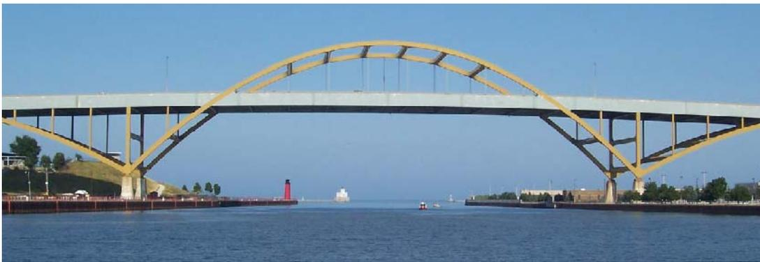
Figure 7-1. Hoan Bridge (Wisconsin, Tied Arch Bridge, Span = 270 + 600 + 270 ft)
