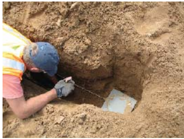
Researchers use pressure plates and MEMS accelerometers to monitor compaction energy
