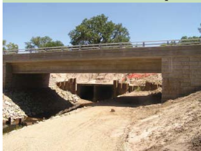
A natural crossing under construction with a trail
