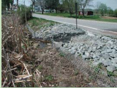
An example of a turtle crossing at construction
