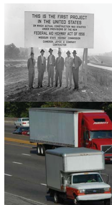
Times have changed. The opening of Missouri Interstate 70 (above) was big news in 1956. Now it's a critical commerce corridor for Midwest multimodal freight movement (below). Photos courtesy of the Missouri DOT
